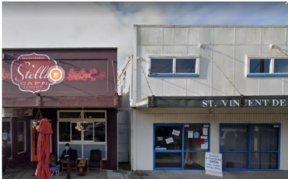
Rooflines hidden behind a parapet
