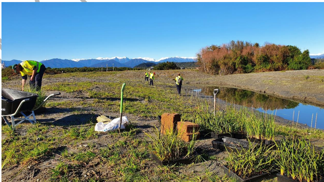
Figure 2: Planting and channel creation activities in progress
