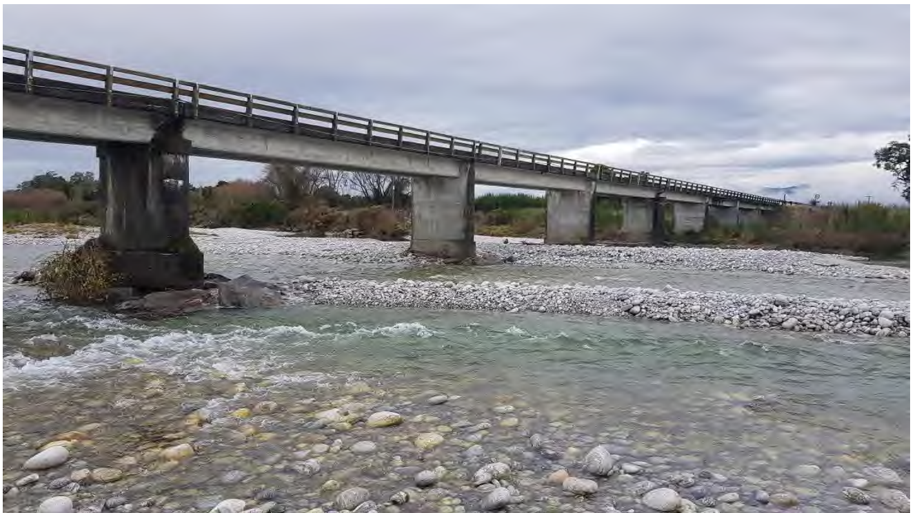
Figure 47: Rough River Bridge
