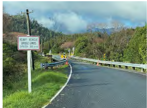
Figure 36: Freight restriction on Tidal Creek No.2 Bridge, Buller District
