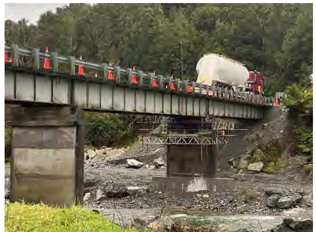
Figure 41: Crooked River No.2 Bridge renewals, Grey District
