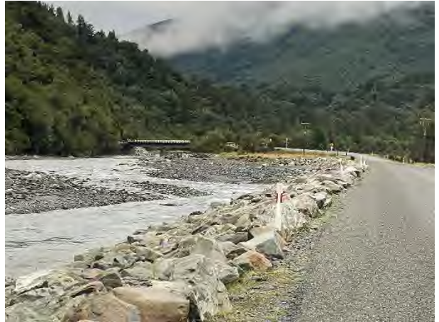
Figure 39: Flood remedial works on Styx River, Westland District
