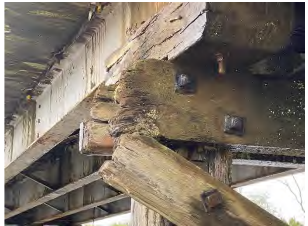
Figure 40: Moonlight Creek Bridge, funded for condition-based replacement (PGF)
