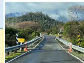
Tidal Creek No.2 Bridge
