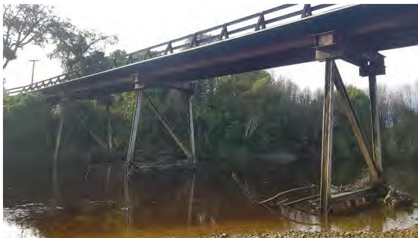
Figure 48: Little Wanganui Bridge
