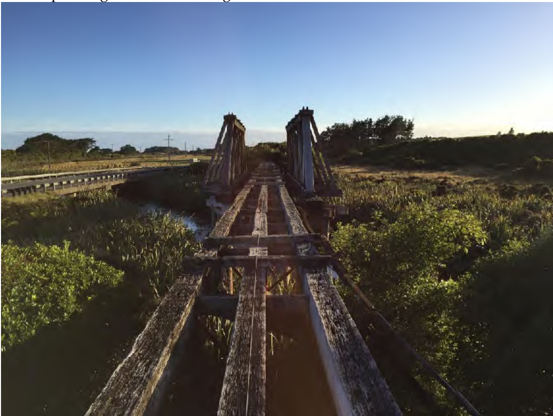
Mahinapua Alignment – Rail Bridge
