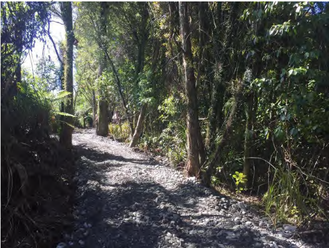
Taramakau Cycle Trail Construction
