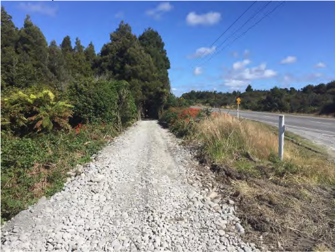
Taramakau Cycle Trail Construction
