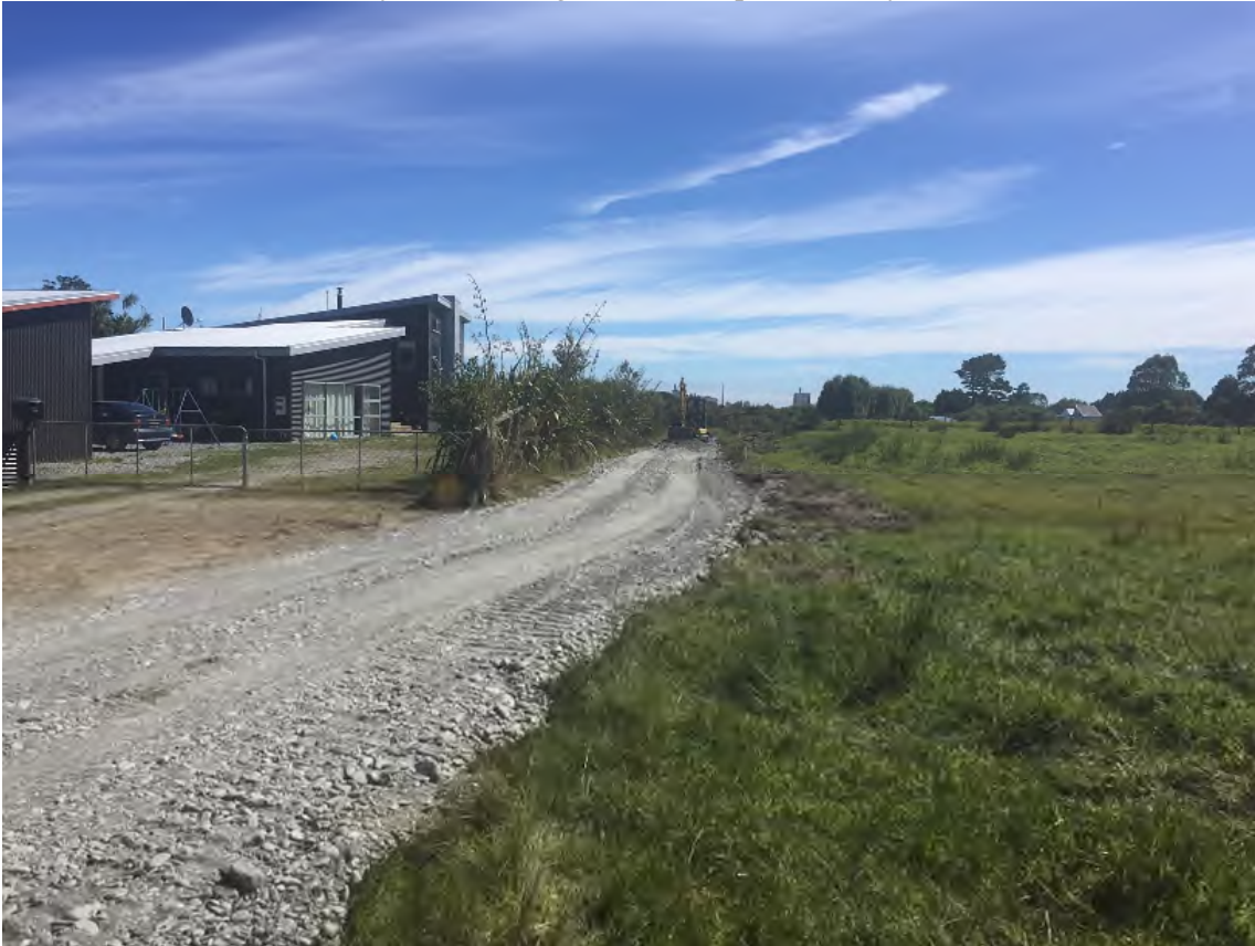
Hokitika-Kaniere Tramway fence realignment and preliminary access
