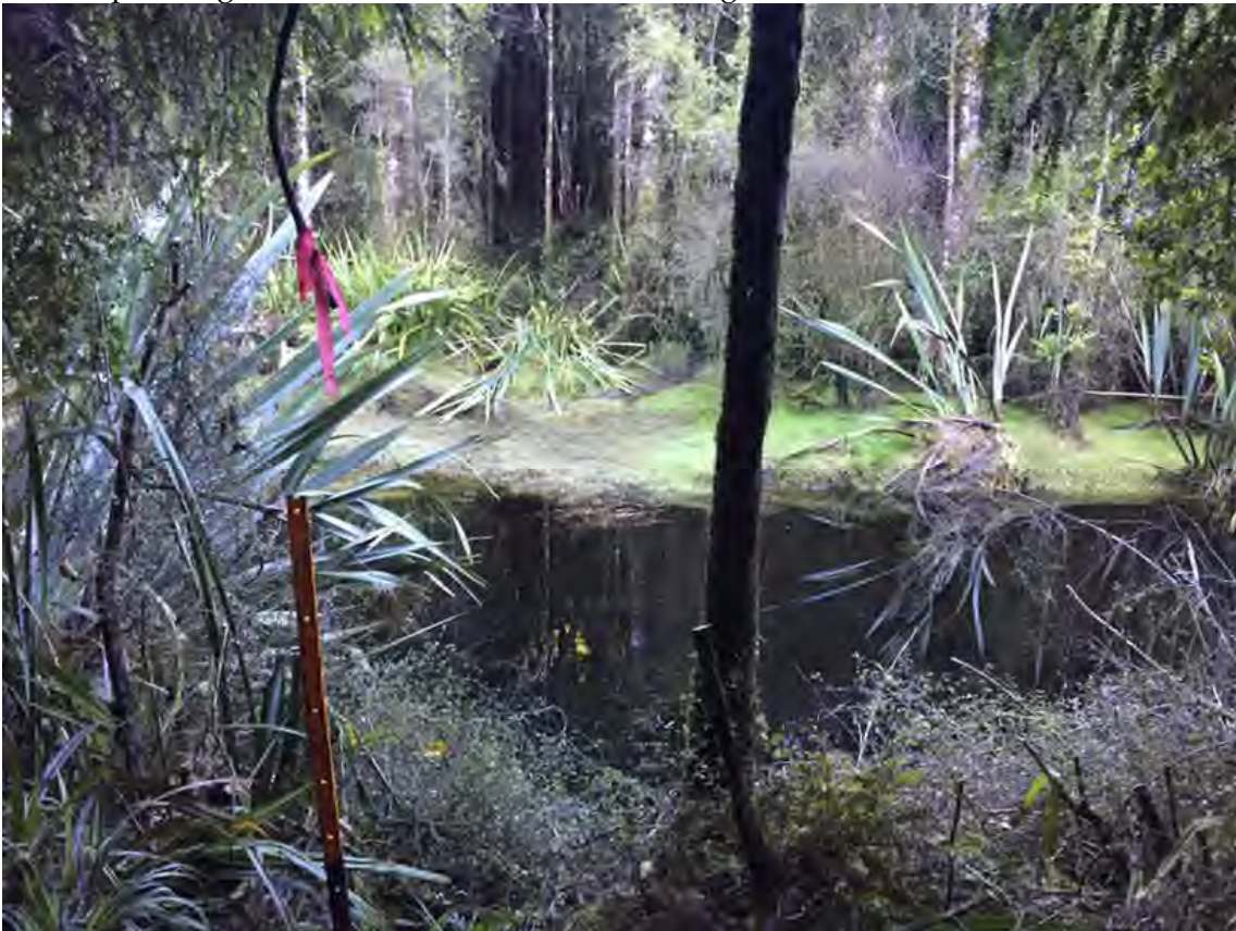
Mahinapua Alignment – Lake Tarleton outfall bridge site
