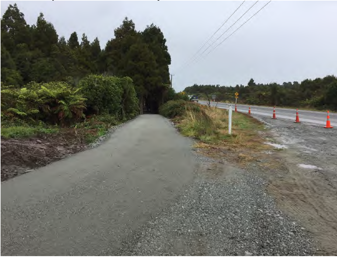
Taramakau Cycle Trail Construction completed
