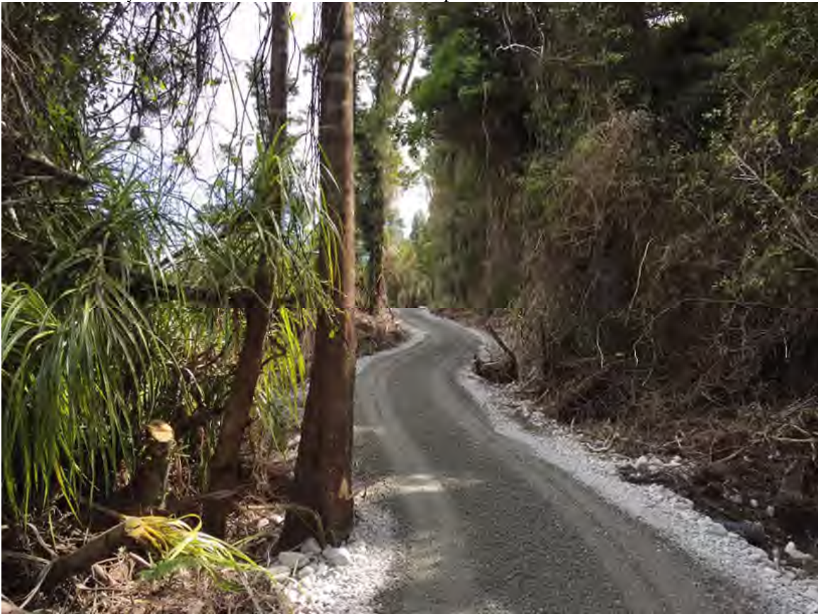
Taramakau Cycle Trail Construction – near completion
