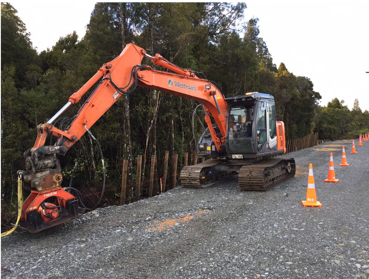
Taramakau realignment by NZTA (Retaining wall posts)
