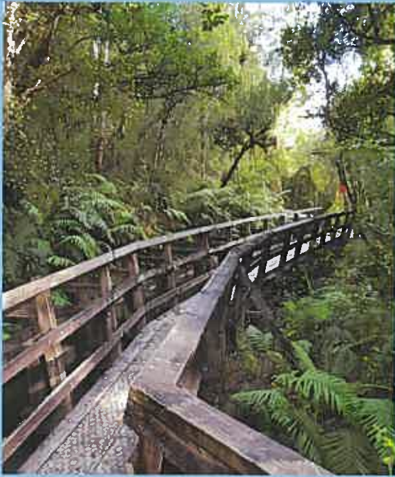
Narrow curved bridge
