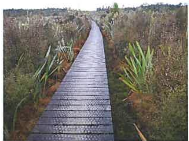
Figure 10: Narrow DoC elevated boardwalk near Lake Mahinapua.
