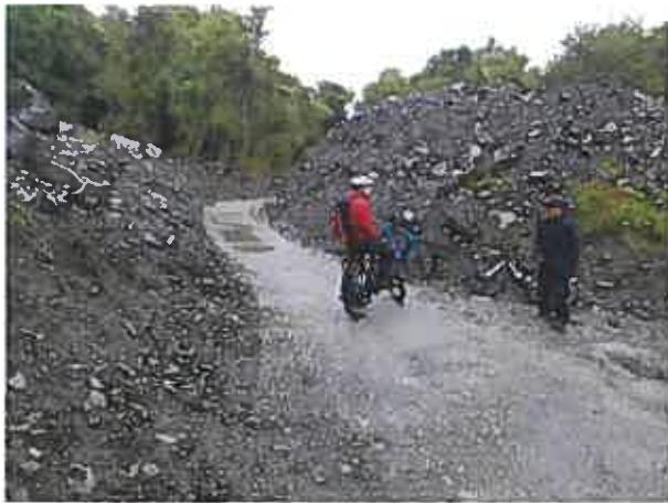
Figure 7: Recent clearing of a March 2019 debris flow to reopen cycle access. Debris flowed downhill from left to right. Photo west of Cowboy Paradise.
