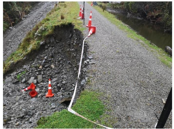
Figure 8: Flooding caused the diversion of river water behind an embankment that subsequently overtopped and eroded the downstream side. Photo west of Cowboy Paradise.
