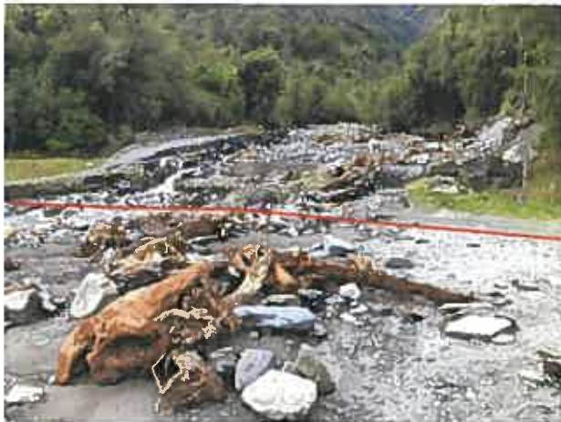
Figure 3: Weir AW2 crossing following March flood damage. Red line shows route of cycle track. Photo supplied by D. Inwood, dated 30 March 2019.
