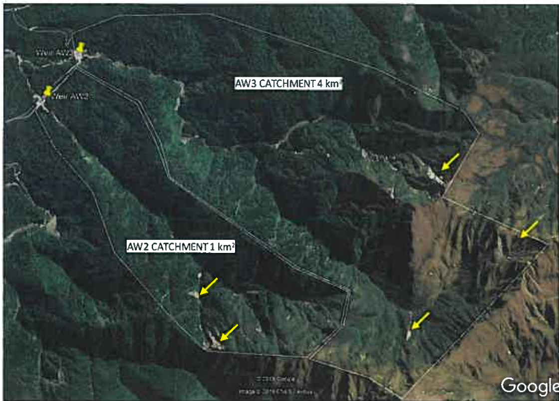
Figure 6: The catchment upstream of the WCWT above weir AW2 and AW3 showing numerous slope failures (yellow arrows). Photo Google Earth (taken 3-02-2019).
