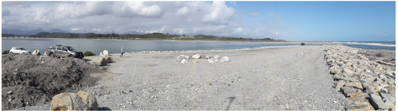
Base levels, fill and rock edging to car park
