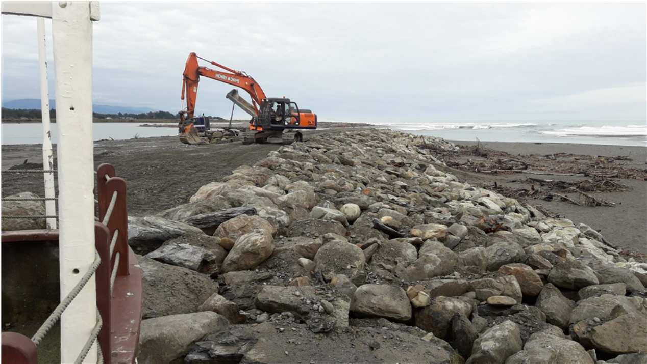
1m high rock protection installation
