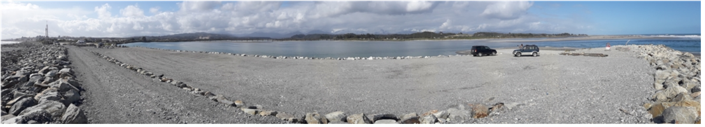
Base levels, fill and rock edging to car park
