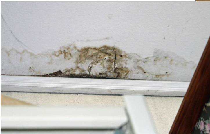
Roof leaks
