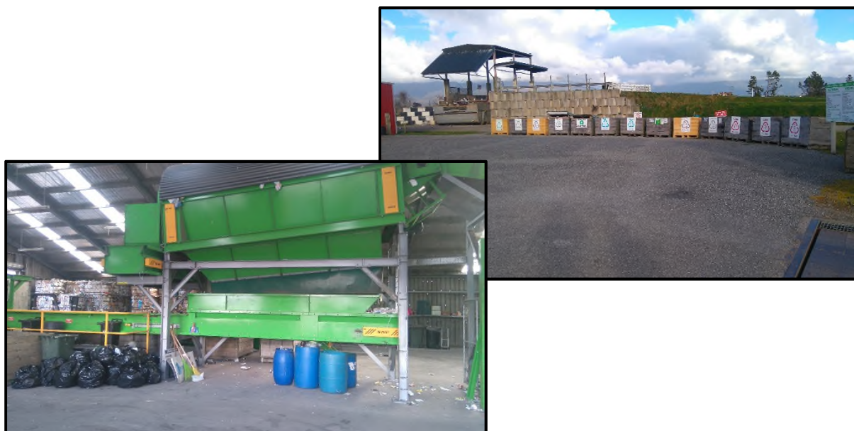
Figure 8: Westport Transfer Station - Drop-off area and MRF
