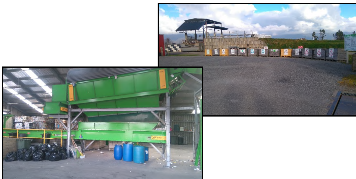
Figure 7: Westport Transfer Station - Drop-off area and MRF
