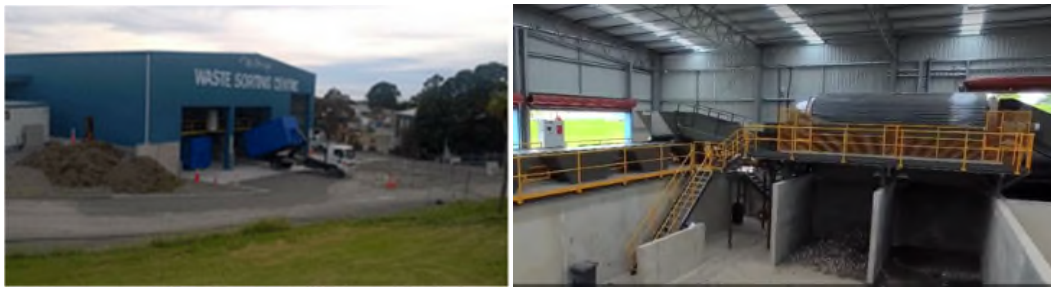
Figure 20 Marlborough Waste Sorting Centre 29
